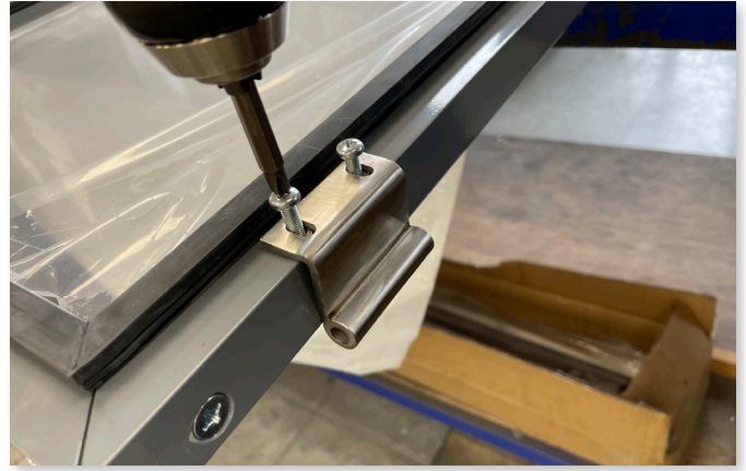
STEP 4 REMOVE SCREWS AND HINGES FROM DOOR
