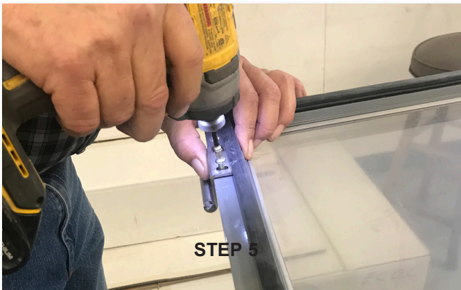
STEP 5 INSTALL UNIVERSAL D-HINGES ON THE DOOR (DO NOT OVER- TIGHTEN)
